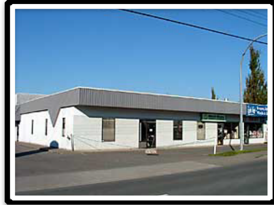
Front of Building
