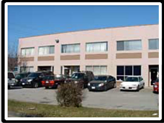
Front of Building
